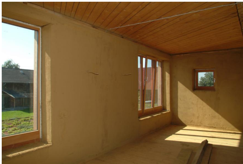
Figure 27 .Earth plaster of straw bale building
